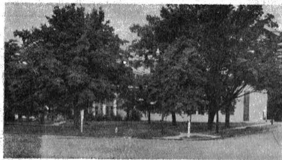
New Addition To Colbert County Court House
